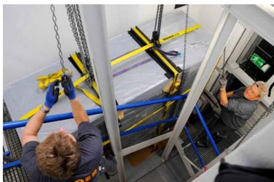
*Fig.3: The XeCl laser (Coherent, Lambda SX) inside the staircase leading to the lidar laboratory in the top floor of UFS*
