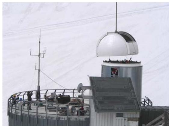
*Fig.4: Assembly of the receiver cabinet on the top platform of UFS: Here, the astronomical dome is delivered as the last component by a big double-rotor helicopter.*
